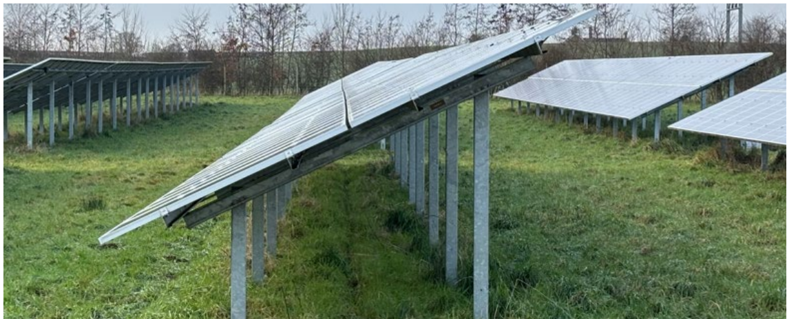
Plate 11-42 Solar PV Arrays Showing Gaps Between PV panels
