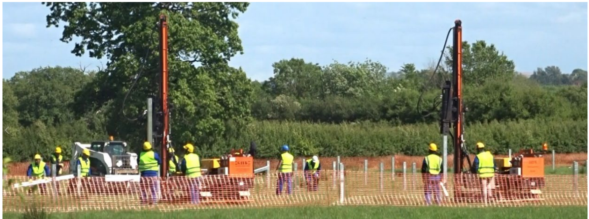
Plate 11-27 Mounting Structure Piles being Installed
